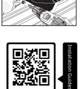
Note: Properly installed the base with Master Seal® Bonded Washers and fasteners. Fasteners should be 1" - 1-1/2" apart around the entire base for a tight secure seal
